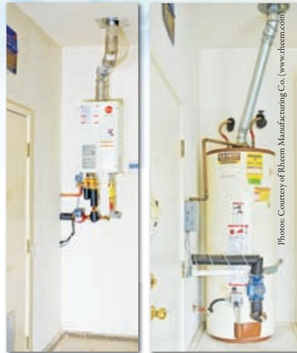
*These photos illustrate the difference in space requirements for a tank-type water heater versus a tankless.*
